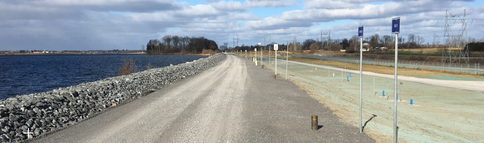
Waba Dam Rehabilitation Project
