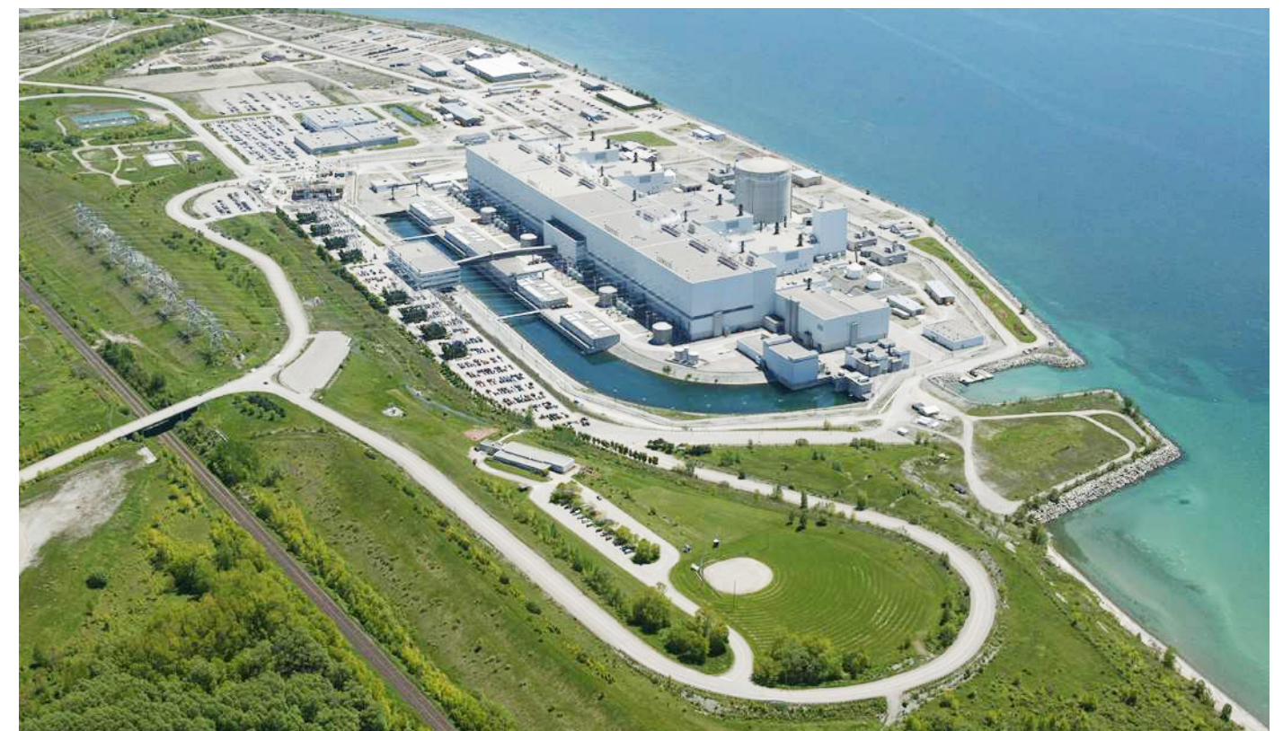
Photo courtesy of Ontario Power Generation
