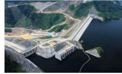
Bakun Dam, 2,400MW
