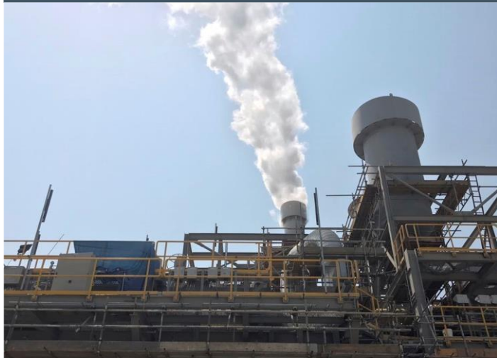
Al Taweelah Alumina Power and Steam
