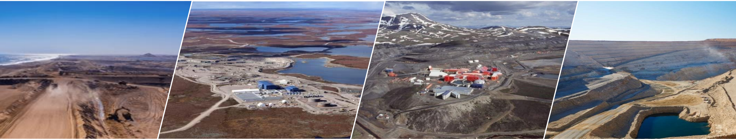
100% Renewable Power Mine, Namdeb Mine (Namibia)
