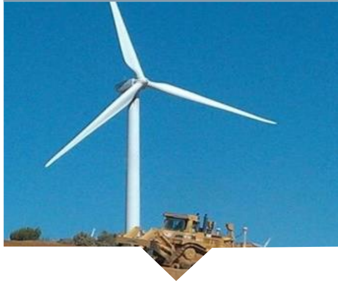
Coram 102MW Wind Farm
