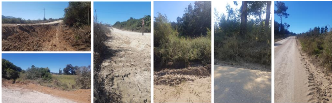
Figure 5: Various examples of the inadequate side drainage along the DR 1797 Road
