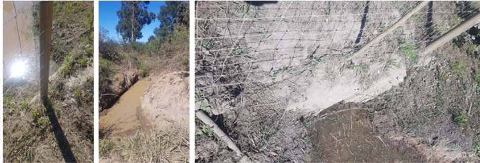
Figure 2-7: Blocked minor culverts
