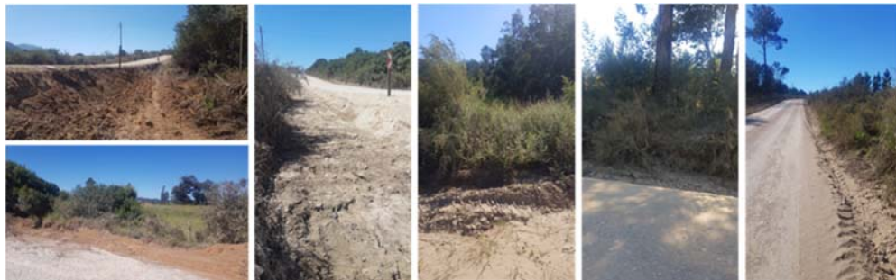
Figure 2-5: Various examples of the inadequate side drainage along the DR 1797
