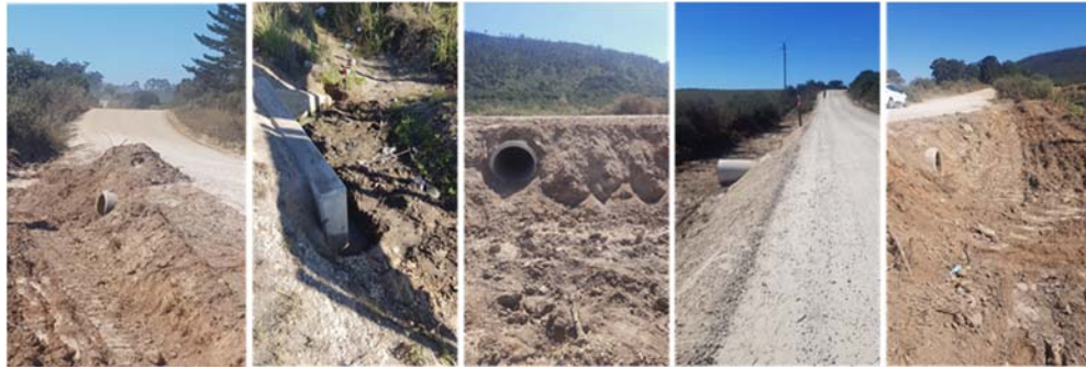
Figure 2-6: Inadequate minor culverts along the DR 1797
