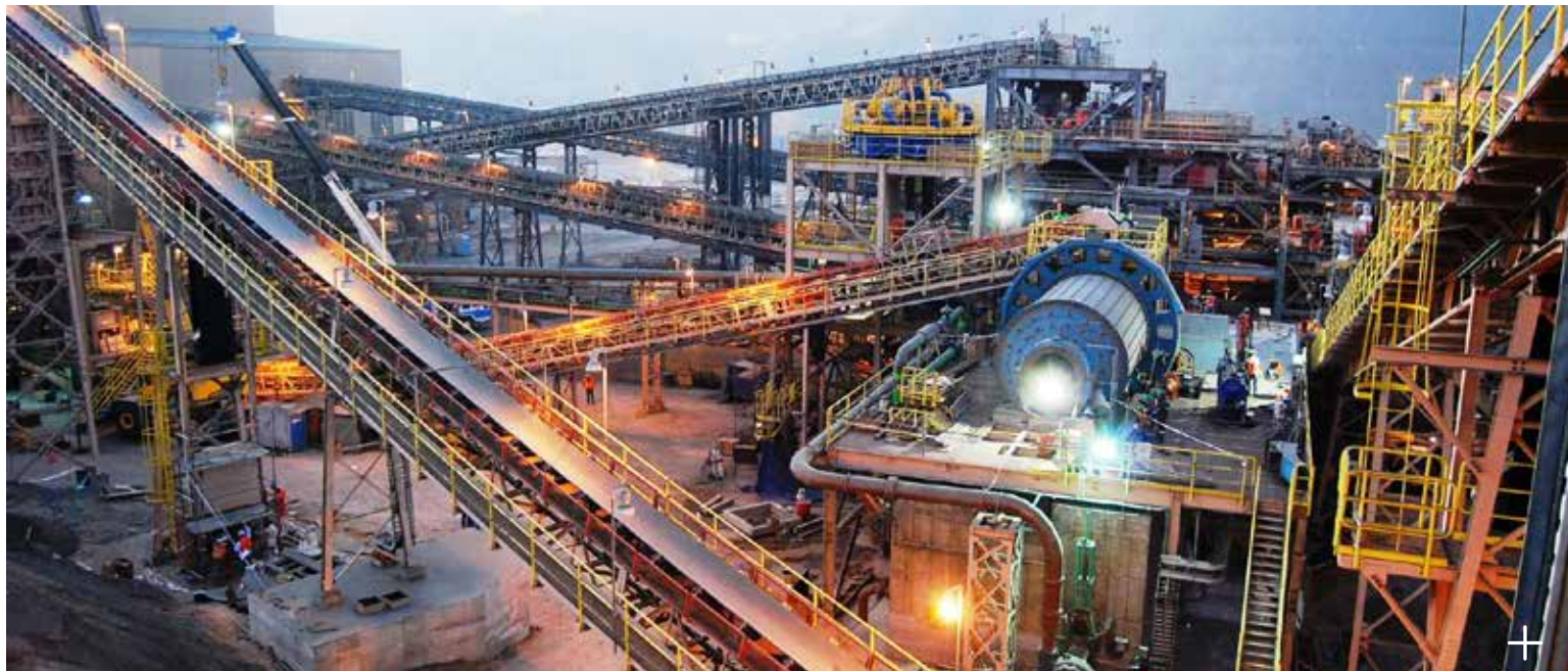
Hatch provided EPCM services for Freeport McMoRan's 300 l/s seawater desalination plant and conveyance system to supply process water to the Candelaria facilities.
