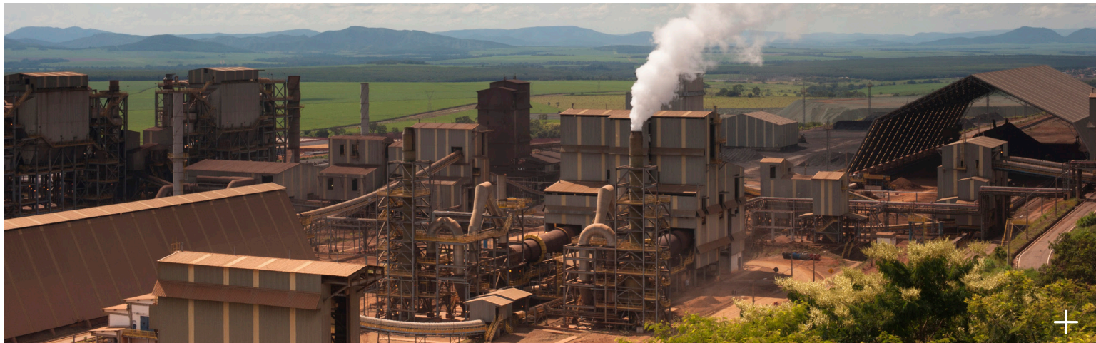
At Barro Alto, two 81 MW rectangular FeNi electric furnaces were upgraded to improve performance at the smelter and reduce the operating risks of the existing furnaces
