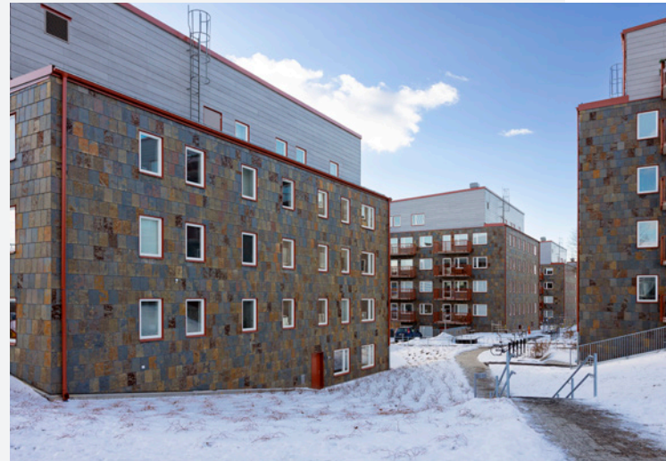
Residential tower blocks in Kållerød, Gothenburg
