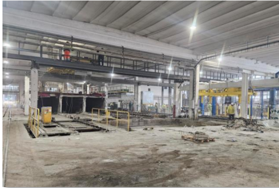
Week 45 – Construction ongoing
