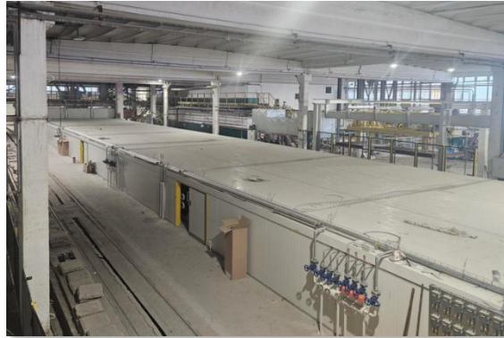
Week 53 – Precuring chamber - ready
