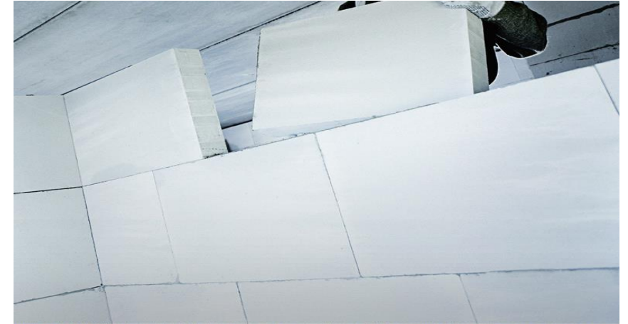
Partition walls in block of flats
