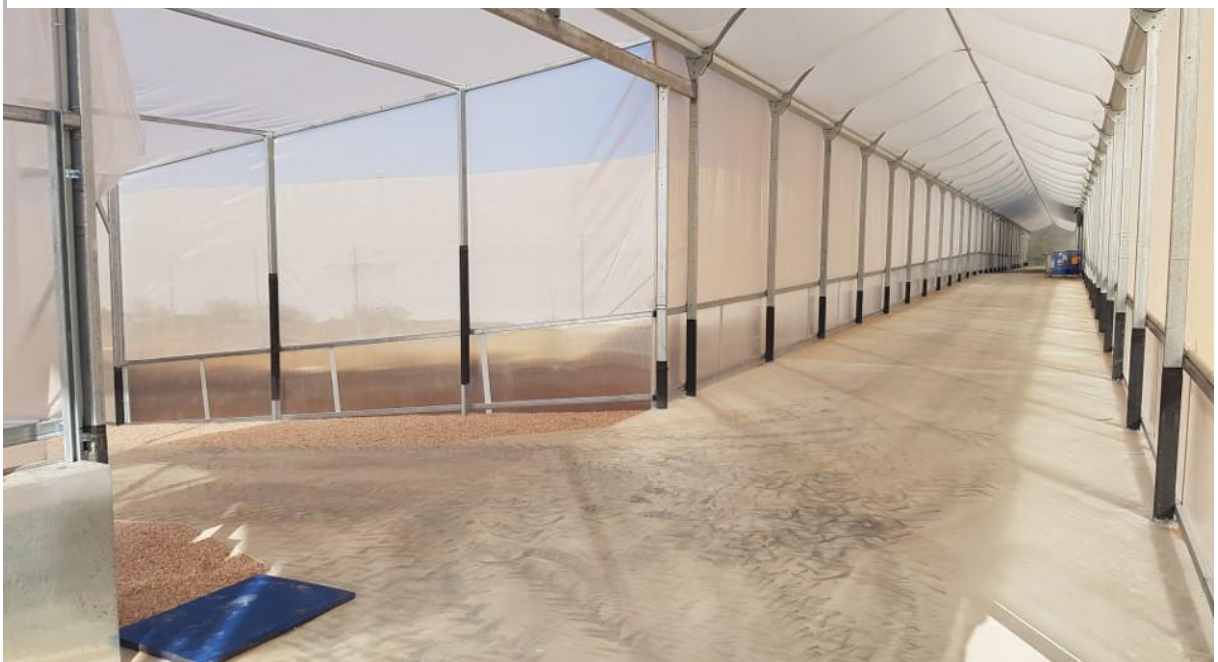
Figure 2 - Atrium connecting new house to existing structures
