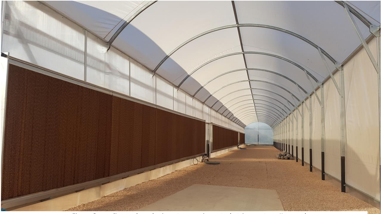
Figure 3 - cooling pads under insect screen in central atrium – stage II screenhouse will be attached to right of this picture
