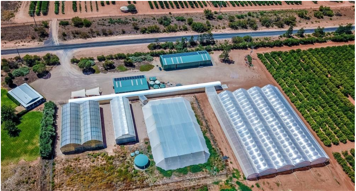
Figure 1- New structure on right of picture – existing shadehouse (centre) will be removed to make way for Stage II development
