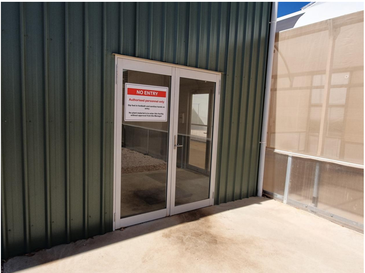
Figure 4 - positive pressure insect lock – all personnel enter through this vestibule
