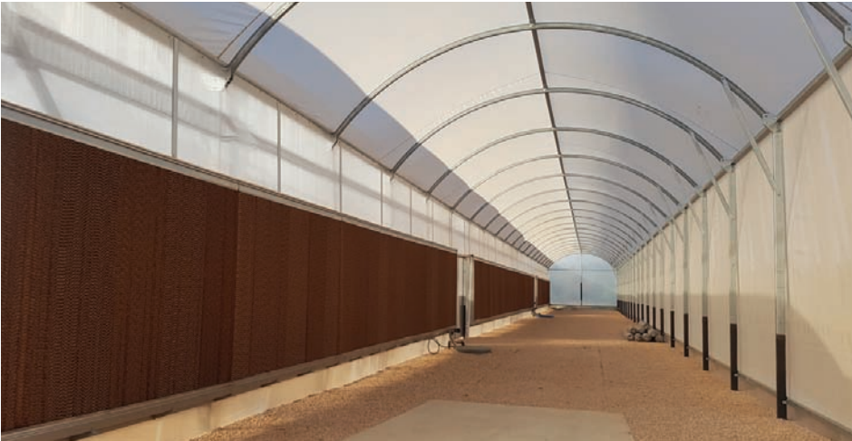
Cooling pads in the new facility.
