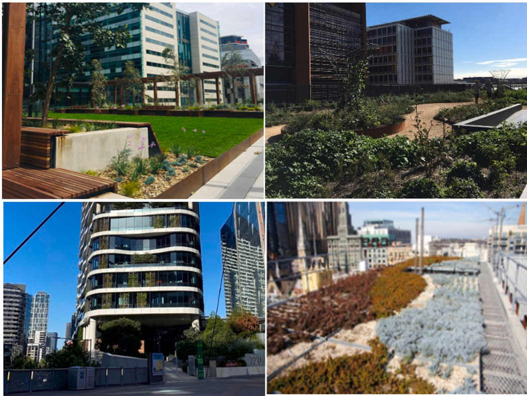
Fig. 1. Selected images of green roofs and facades in Sydney and Melbourne.
