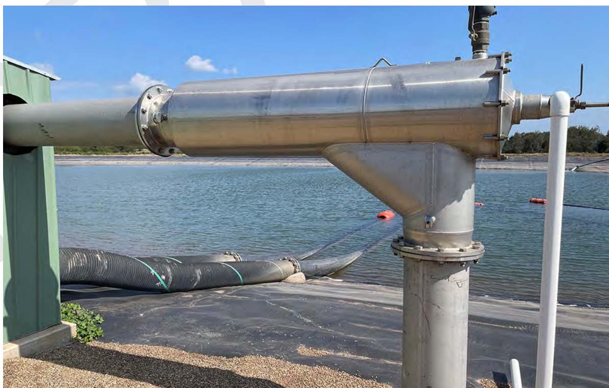
Figure 58. Using coarse filtration and frequent backflushing minimises the sediment and reduces the microbial population in irrigation water.
