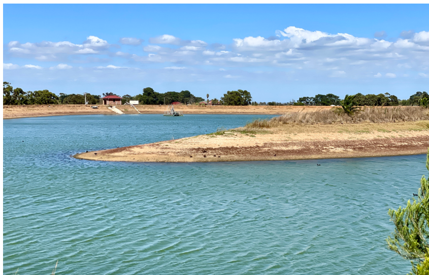
Figure 2: On-farm dam used for storing irrigation water, generally pumped from surface water sources such as rivers and creeks.
