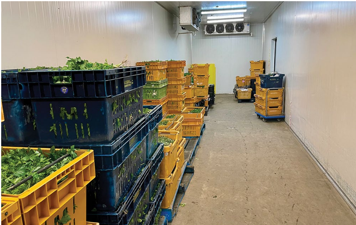
Figure 43. A cold storage facility used for cooling of harvested produce on a small-scale farm.
