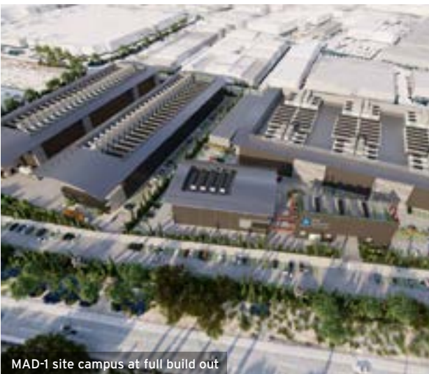
MAD-1 site campus at full build out
