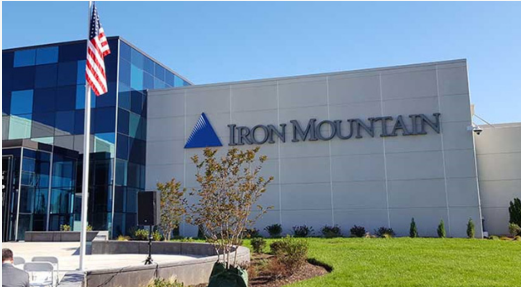
Iron Mountain's data center in Manassas, Virginia
