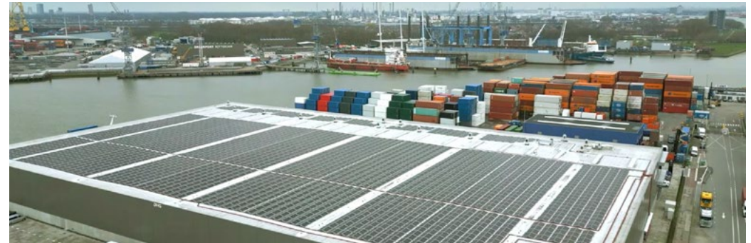
In a step towards complete decarbonization, Iron Mountain Data Centers recently signed a solar Power Purchase Agreement with Sunrock, who are expanding a 4MW solar rooftop array on warehouses in the Port of Rotterdam: watch video here
