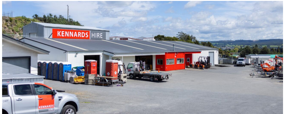
1. Tauhara Power Station project site, 2. Kennards Hire new branch Taupo,
