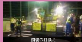
舗装の打換え
