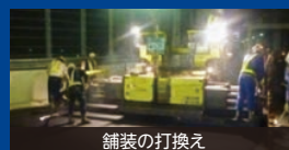
舗装の打換え
