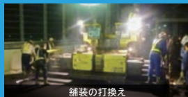
舗装の打換え
