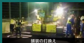
舗装の打換え
