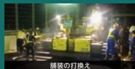
舗装の打換え
