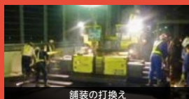
舗装の打換え
