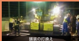
舗装の打換え
