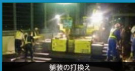
舗装の打換え
