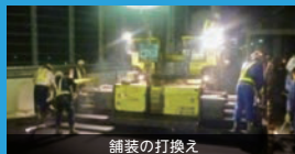
舗装の打換え
