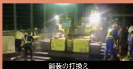
舗装の打換え
