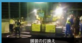
舗装の打換え
