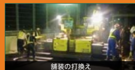
舗装の打換え
