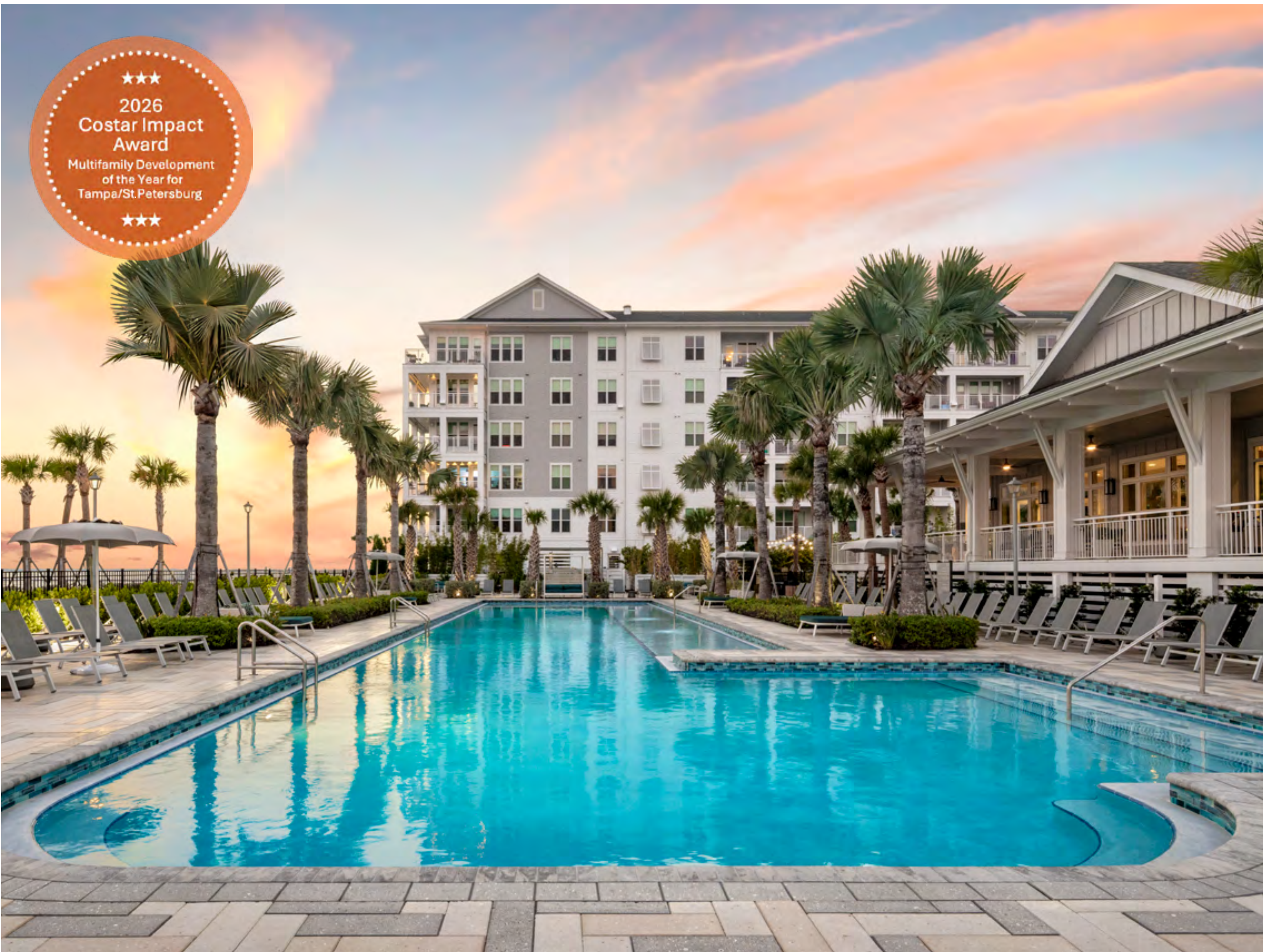
MAA Breakwater, Tampa, FL
