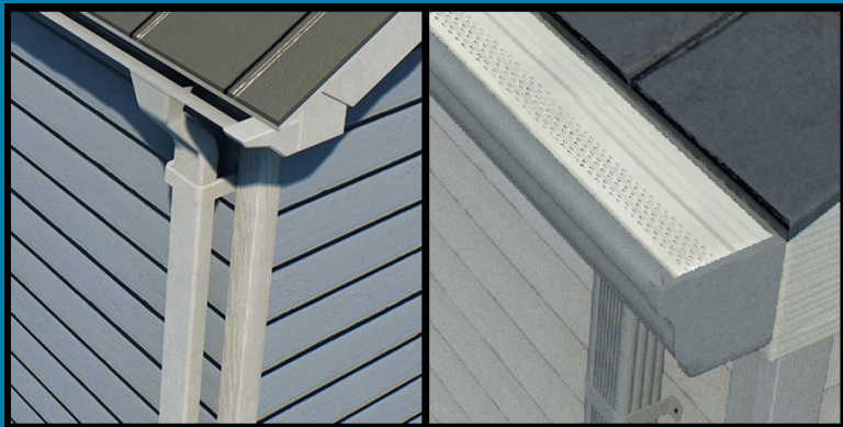
Gutter and downspout (left); gutter with cover (right)
