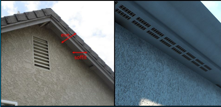
Eaves and soffit (left); eave enclosure (right)
