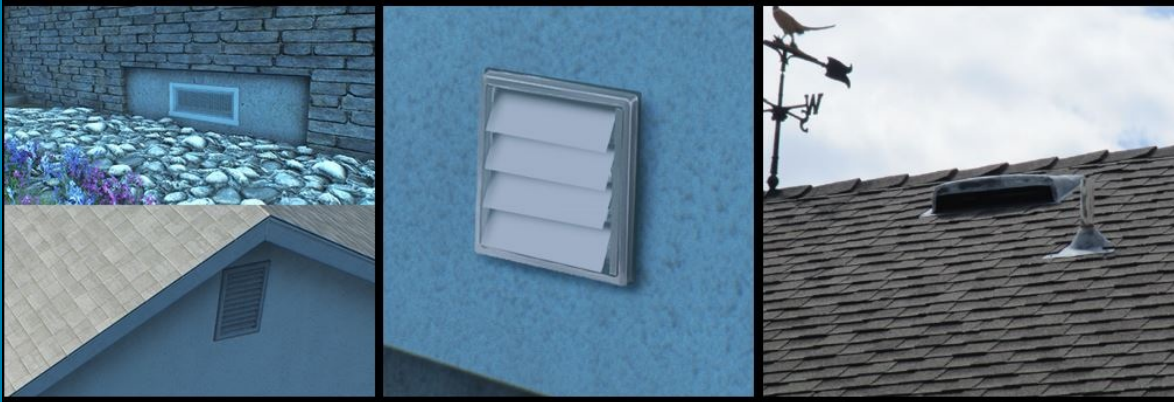
Crawlspace vent (top left), gable end vent (bottom left), dryer vent (middle), roof vents (right)
