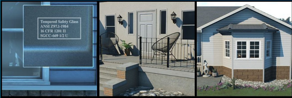
Fire resistant glass (left); exterior door (middle); enclosed bay windows (right)
