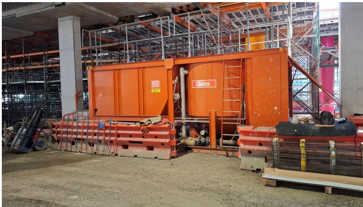
19. Part of the groundwater treatment plant. 25/06/25
