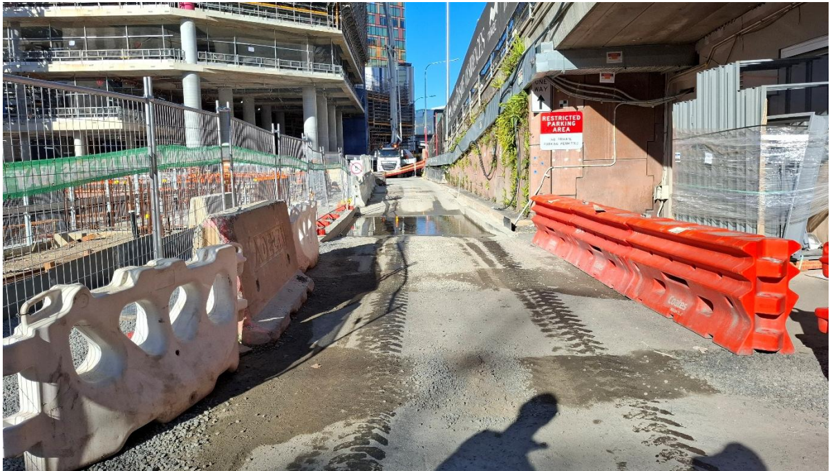
13. Site truck exit with wheel wash and rumble grid. 25/06/25
