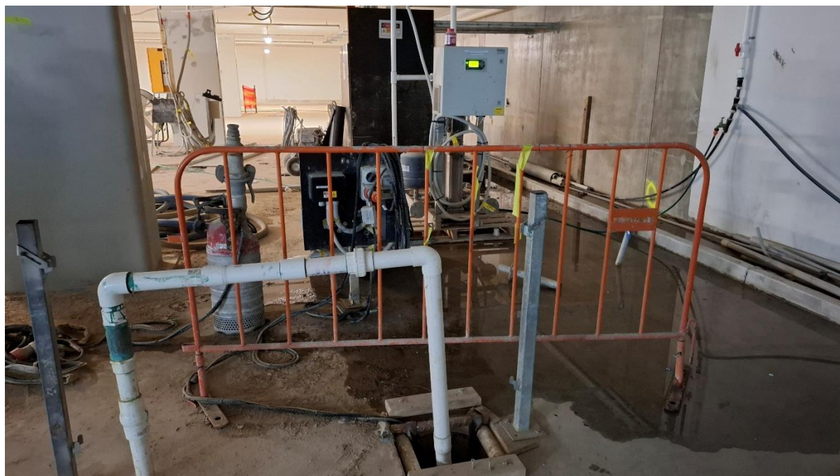
26. Groundwater extraction in the basement. 25/06/25
