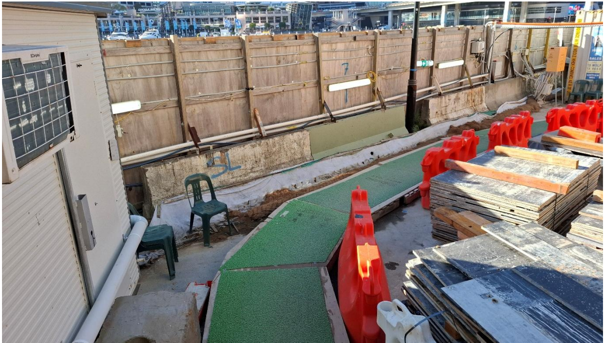
15. Sediment controls inside the eastern hoarding. 25/06/25
