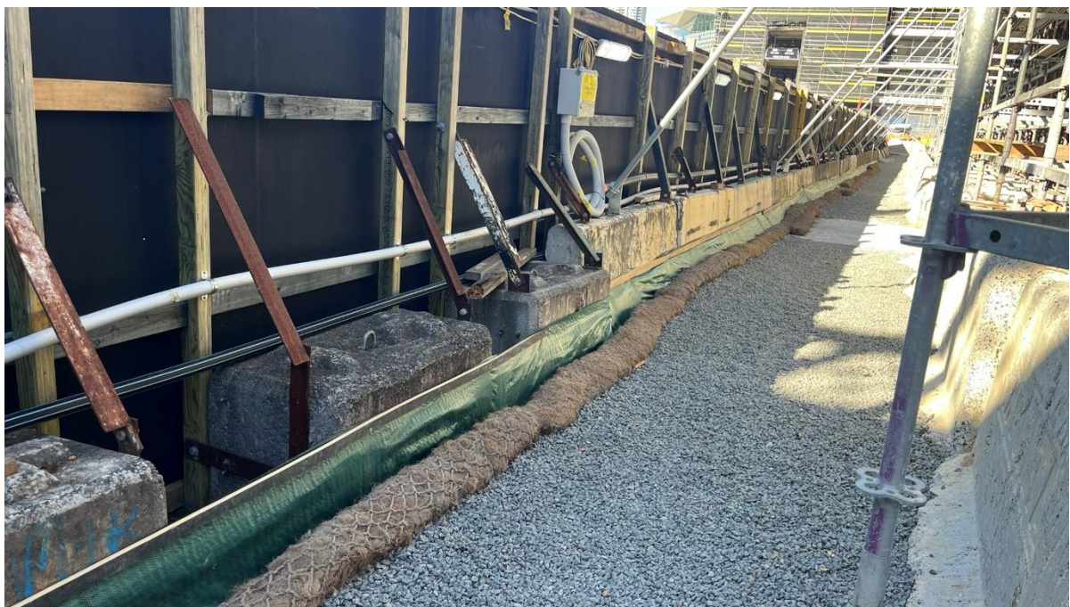
14. Sediment controls inside the eastern hoarding. 25/06/25
