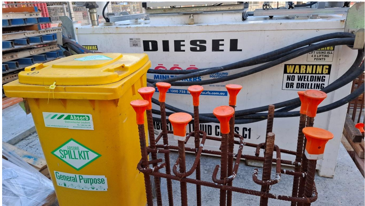
21. Self-bunded Diesel Tank with nearby spill kit. 25/06/25
