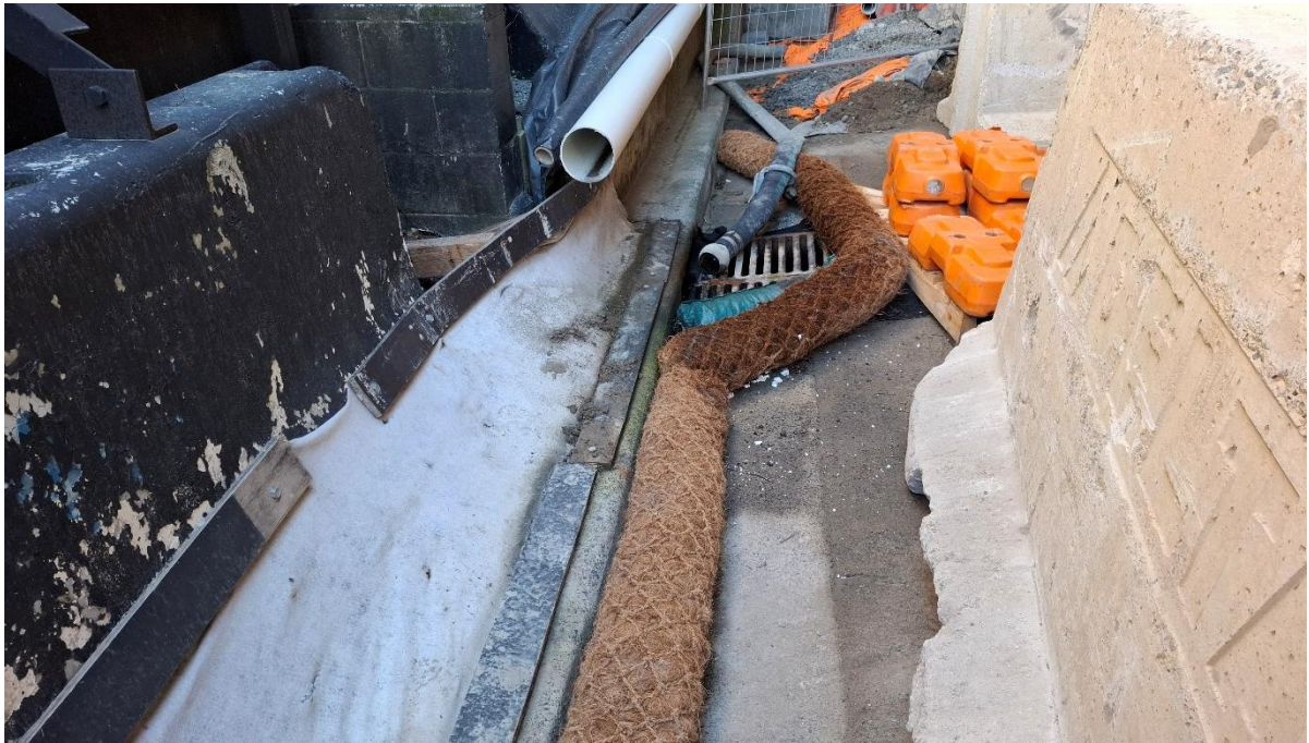
17. Sediment controls around stormwater drain where the groundwater treatment plant discharges. 25/06/25
