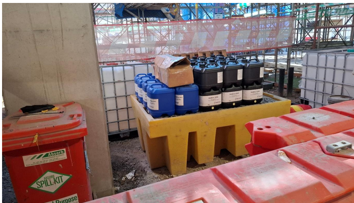
20. Storage of water treatment chemicals on a pallet bund and a nearby spill kit at the groundwater treatment plant. 25/06/25
