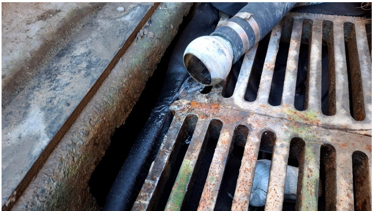
18. Clear groundwater treatment plant discharge. Stormwater drain also has drain guard protection. 25/06/25
