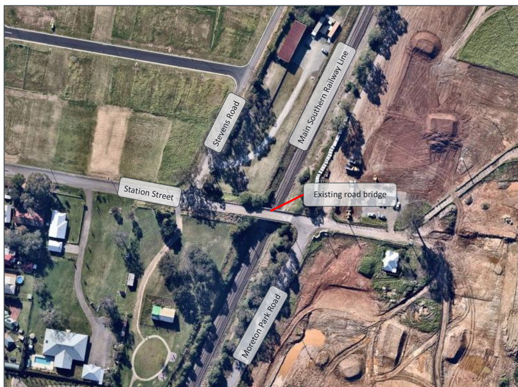
Figure 1-1: Aerial view of the existing road bridge over the Main Southern Railway Line (source: Nearmap, 2022)
