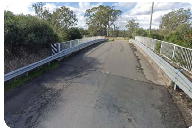
Figure 9: View Looking East at the Vehicular Bridge Source: Google Maps 2021
