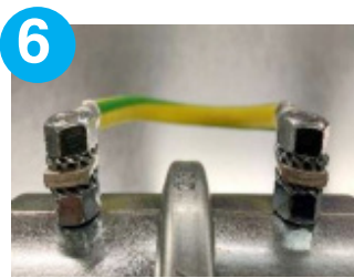
6 Continue with the cable washer and nut and then tight the parts.
