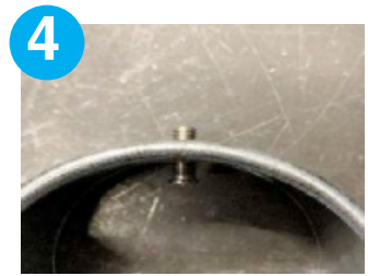
4 Shrew the bolt from inside.
