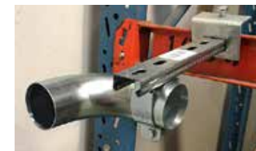
Assembled Beam Clamp with Pipe Clamp holding Bend.
