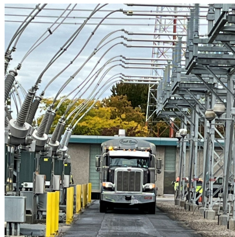
→ NIA 115kV Switchyard Repaving Clearance Check
