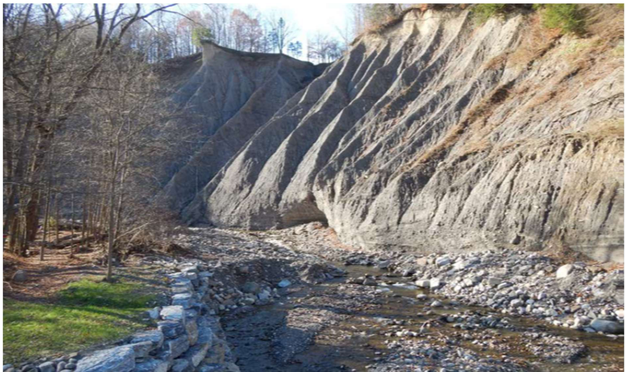
Figure 30. Looking upstream at massive slope failure on Fulmer Creek.
