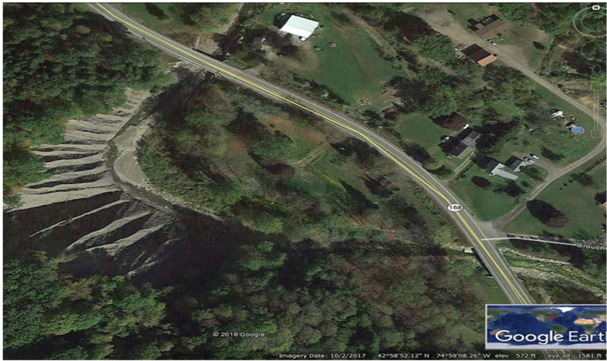
Figure 29. Aerial view of massive slope failure on Fulmer Creek.
