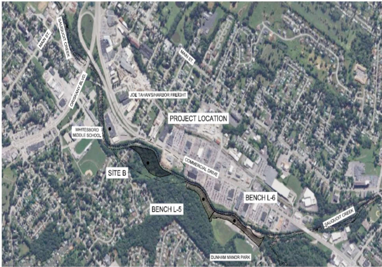
Figure 9. Aerial view of Project 3-Site B along Sauquoit Creek within town of Whitesboro. This project is located just downstream from the floodplains that were restored in Dunham Manor Park.
