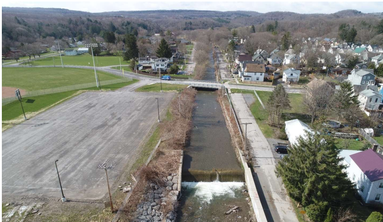
Figure 18 Preconstruction – Aerial view of Steele Creek looking upstream. Remington Arms Company Dam is in the foreground, which causes the channel bed to be raised by as much as 15 feet, contributing to frequent and damaging flooding within the community.
