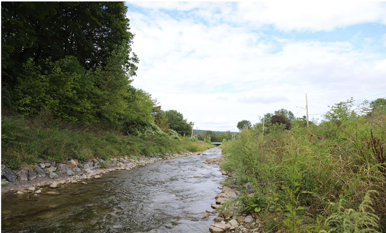
Figure 24. Post construction - View looking downstream on Steele Creek two years after the project was constructed. In-stream features are visible in the channel. The constructed floodplain conveys flood flows during major storm events.
