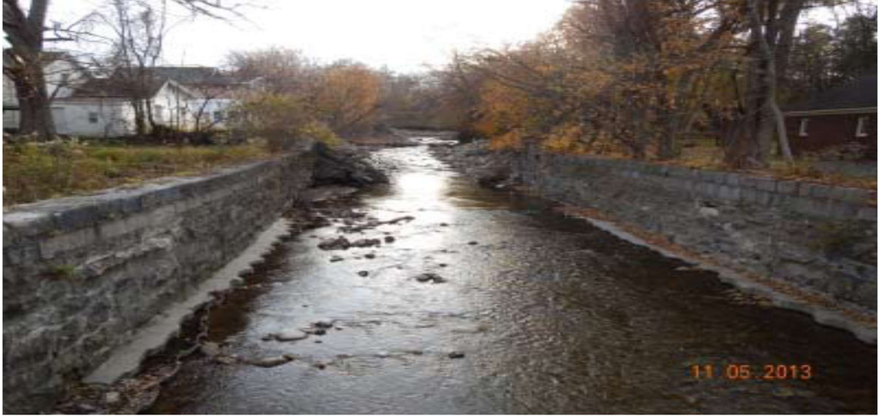
Figure 38. Looking upstream from the Main Street bridge, Moyer Creek is confined by the stone-lined channels before and after crossing Main Street.
