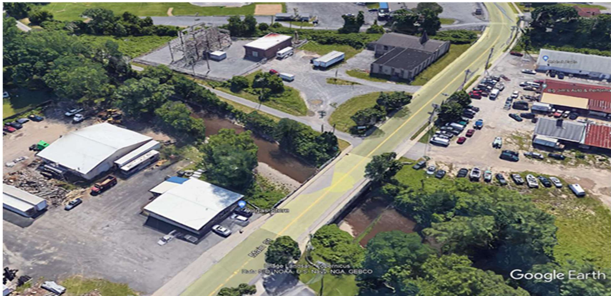
Figure 10. Aerial view of Main Street bridge that will be replaced and upsized by NYSDOT. Please note areas just upstream of this bridge will also be restored to natural floodplains all the way up to State Route 69 bridge.
