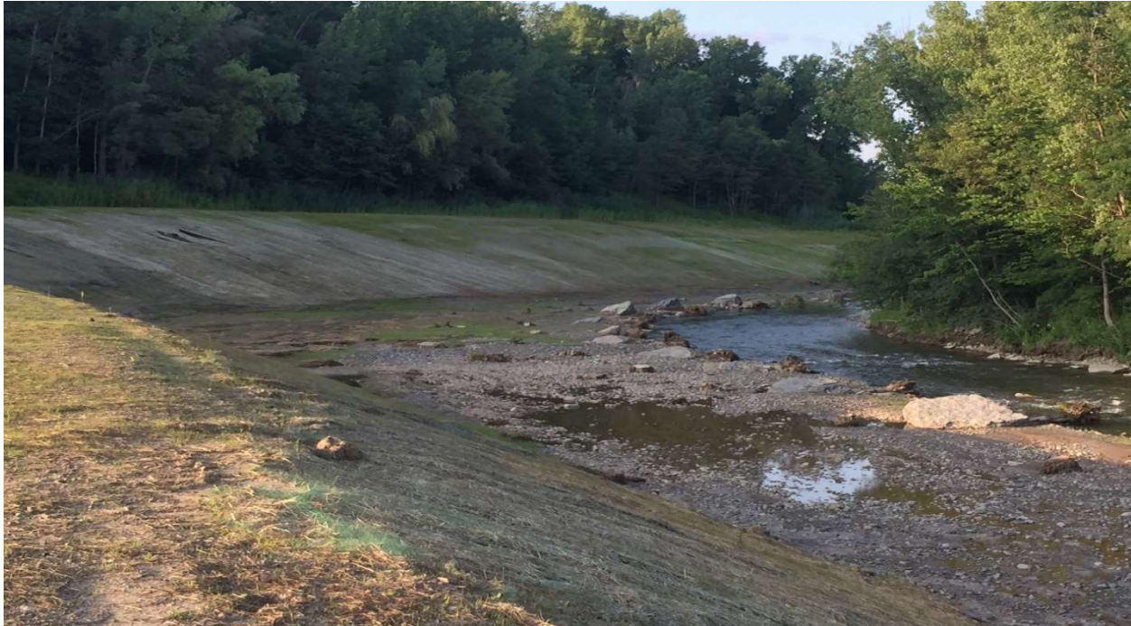
Figure 5. Completed construction of Project 1 within Dunham Manor Park, Town of Whitestown.
