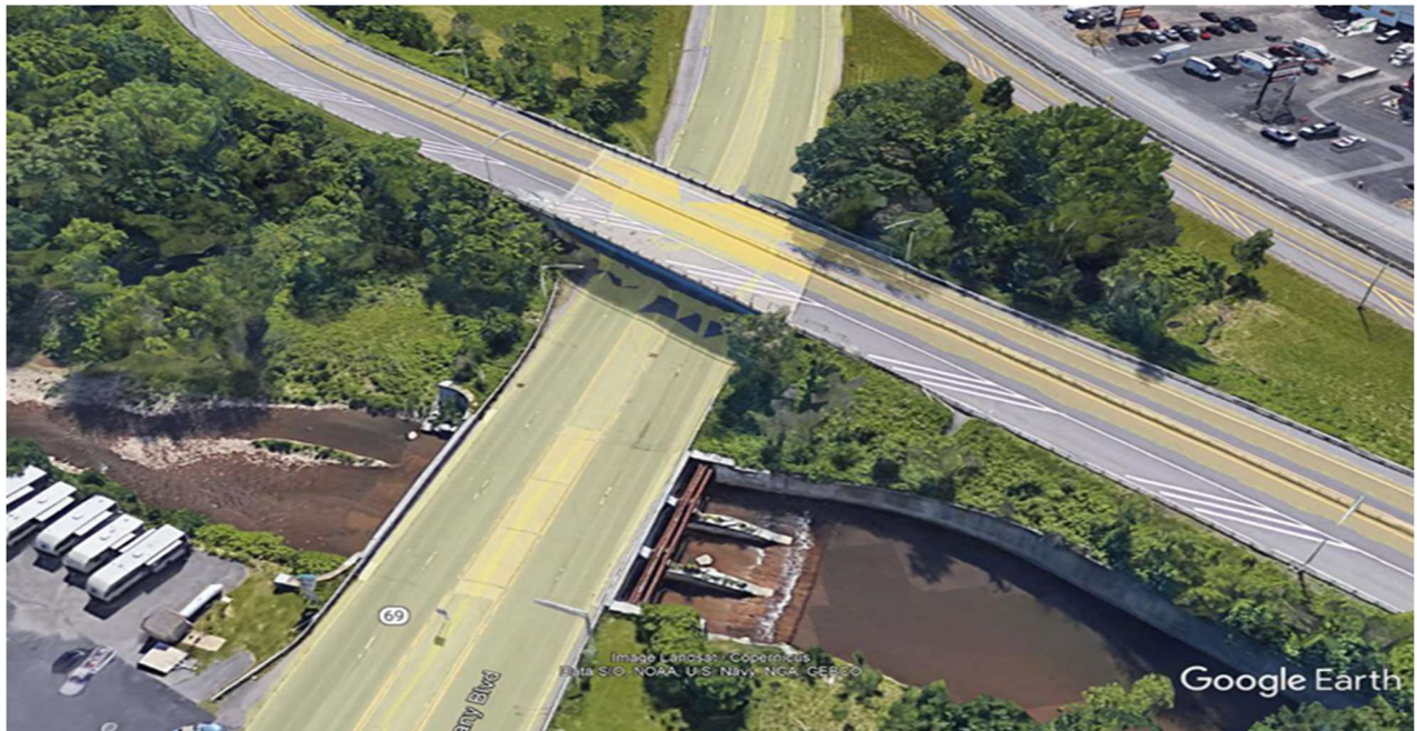
Figure 12. Aerial view of State Route 69 or Oriskany Boulevard Bridge that will be replaced and upsized by NYSDOT.
