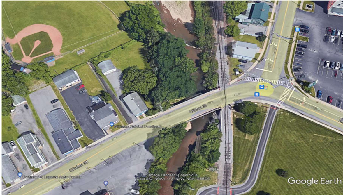
Figure 15. Aerial view of Clinton Street bridge replacement on Sauquoit Creek by the Town of New Hartford.
