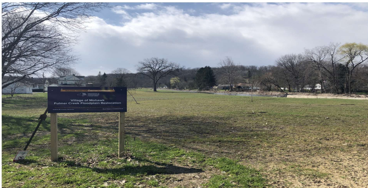
Figure 33. Photo of completed Fulmer Creek floodplain restoration project within Village of Mohawk.
