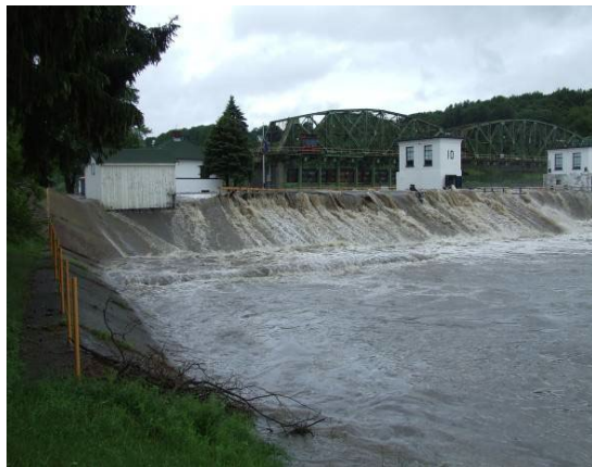
Figure 6: Flow over Spillway
