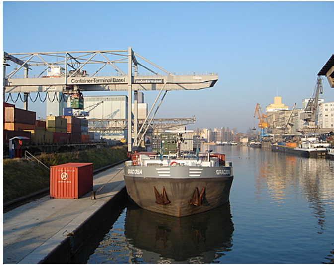
Figure 34: Container Port of Basal Switzerland -- 100,000 TEU per annum, 600 miles, 885 feet above Rotterdam
