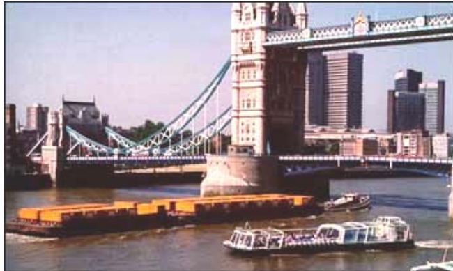
Figure 49: Waste Barge Sharing the Thames with Sight-seers and Tower Bridge
