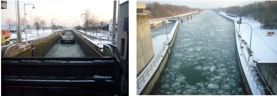
Extreme cold and icing has caused ad-hoc closures of a few days per year.
