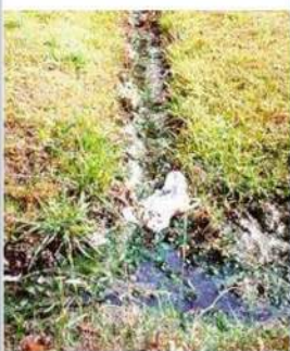
Failing Septic Systems
