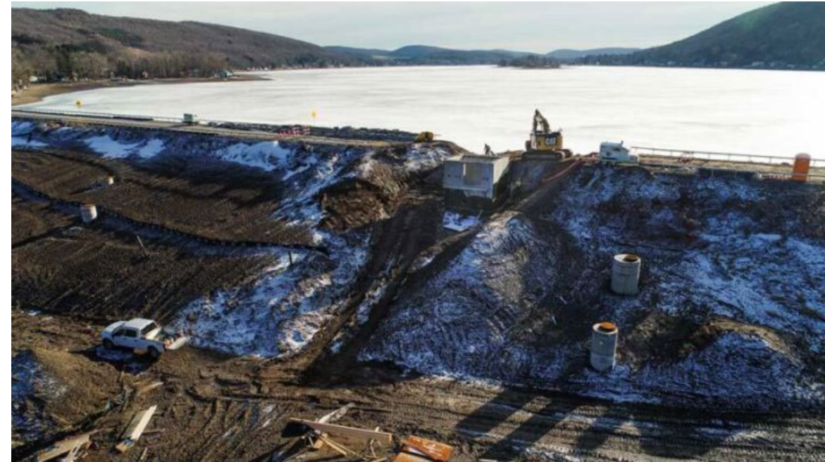
Construction Photo of the DeRuyter Reservoir Dam Rehabilitation Project
