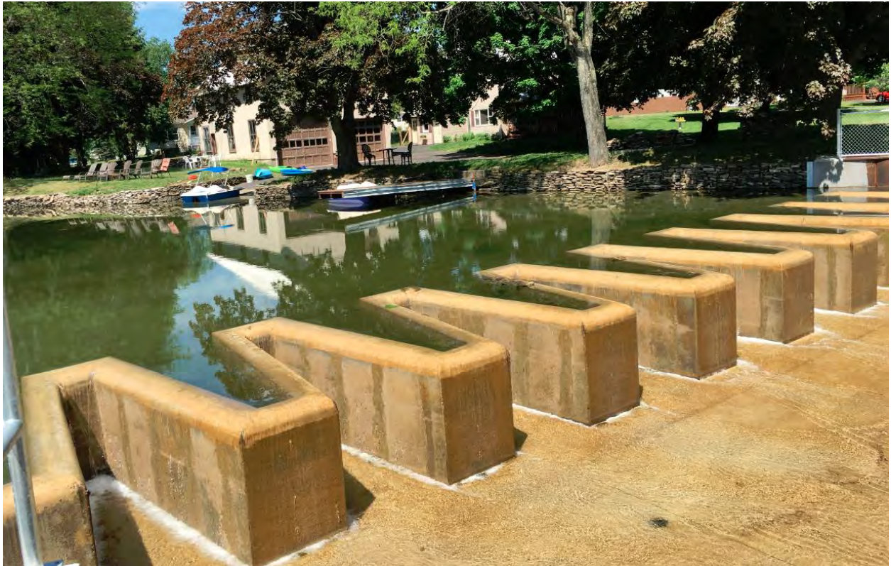
Figure A.2 - Labyrinth Weir
