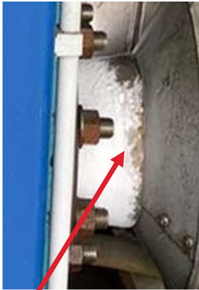
Oil leak, bottom of glycol HX
