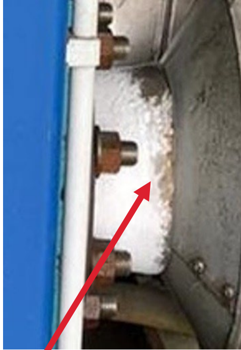
Oil leak, bottom of glycol HX
