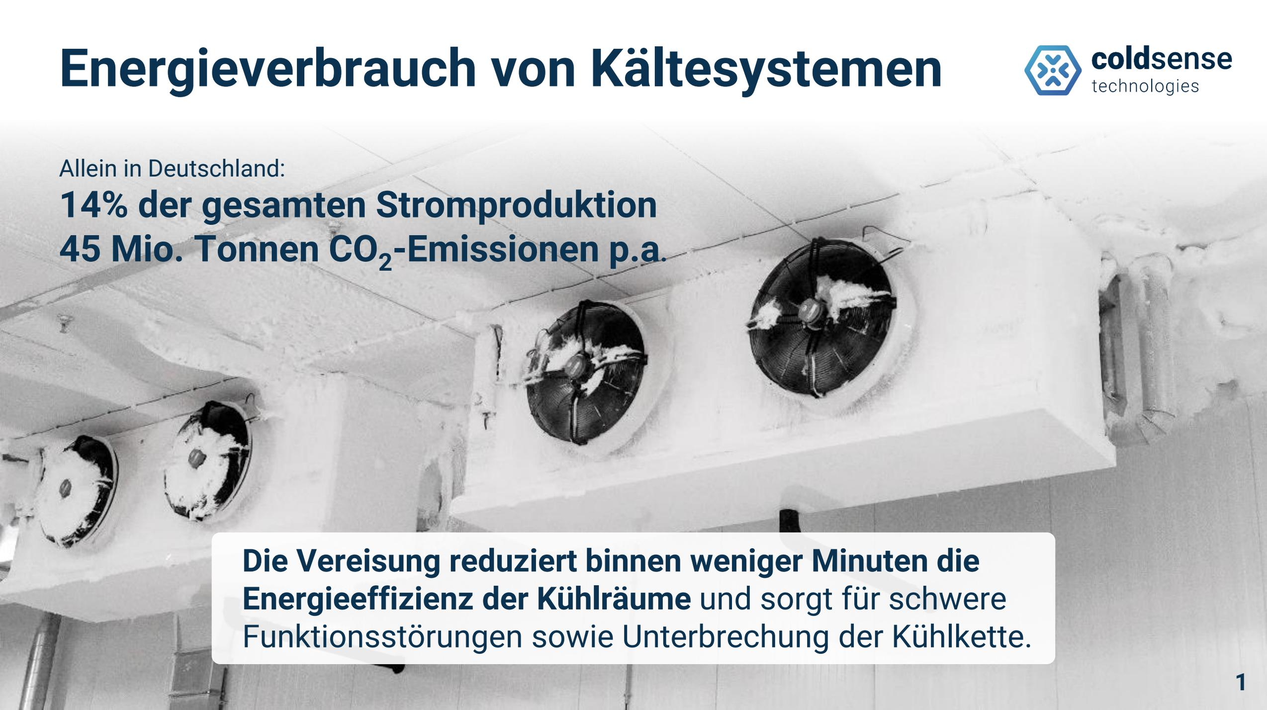
A photograph of a ceiling with several circular fans. The fans are heavily covered in white frost, indicating a significant ice buildup. The ceiling is made of white acoustic tiles.
