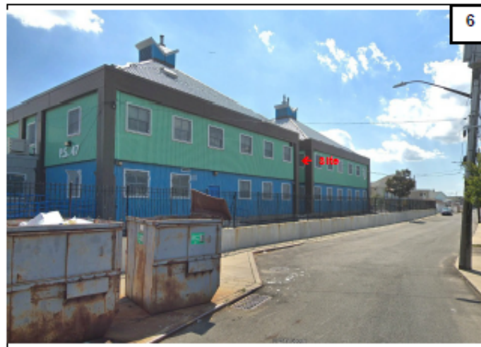
Looking at South on Shad Creek Road
