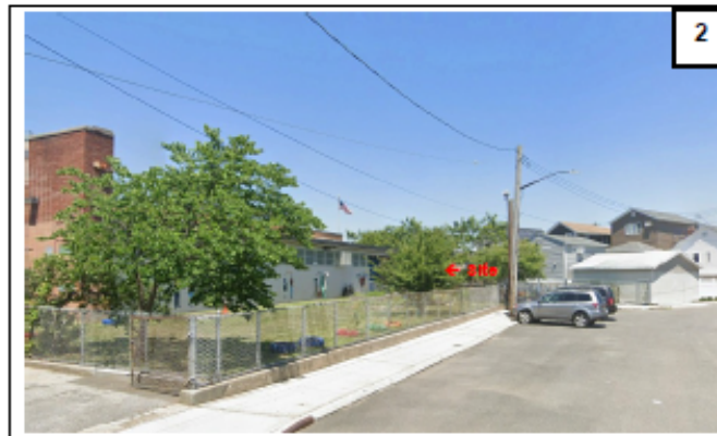
View looking North on Power Road
