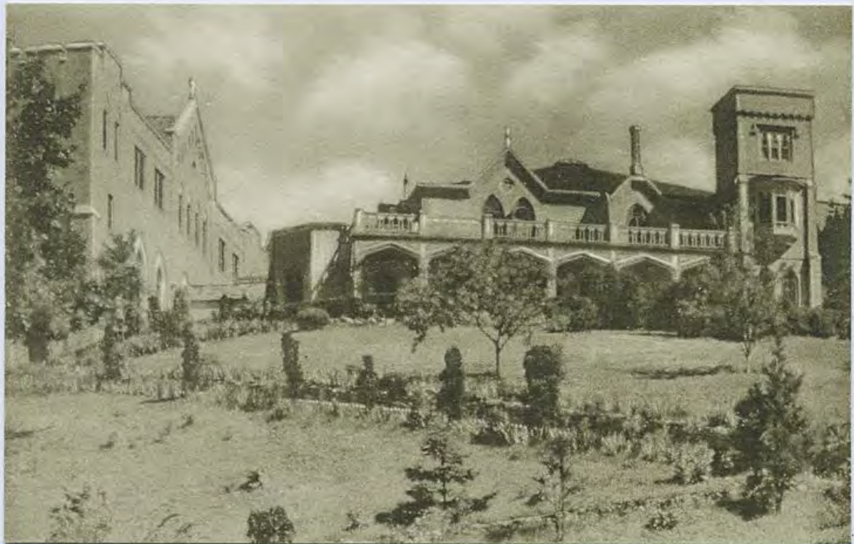
An undated view of the rear of the Villa, showing the wraparound porch that later was rebuilt and enclosed as an extension with a full basement. View looking northwest.
