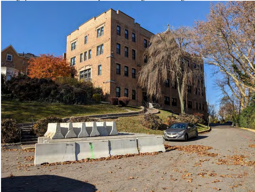
Photograph 6. The former elementary school building, showing its construction into the side of the hill. View looking northwest.
