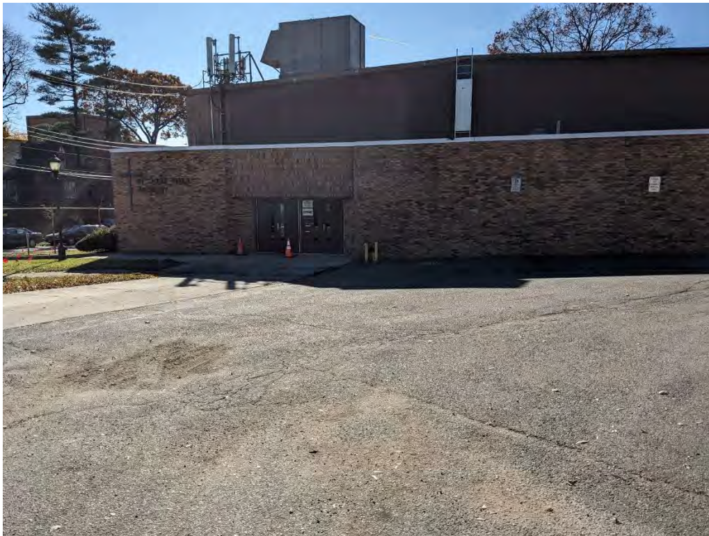
Photograph 12. The former gymnasium building. View looking southeast.
