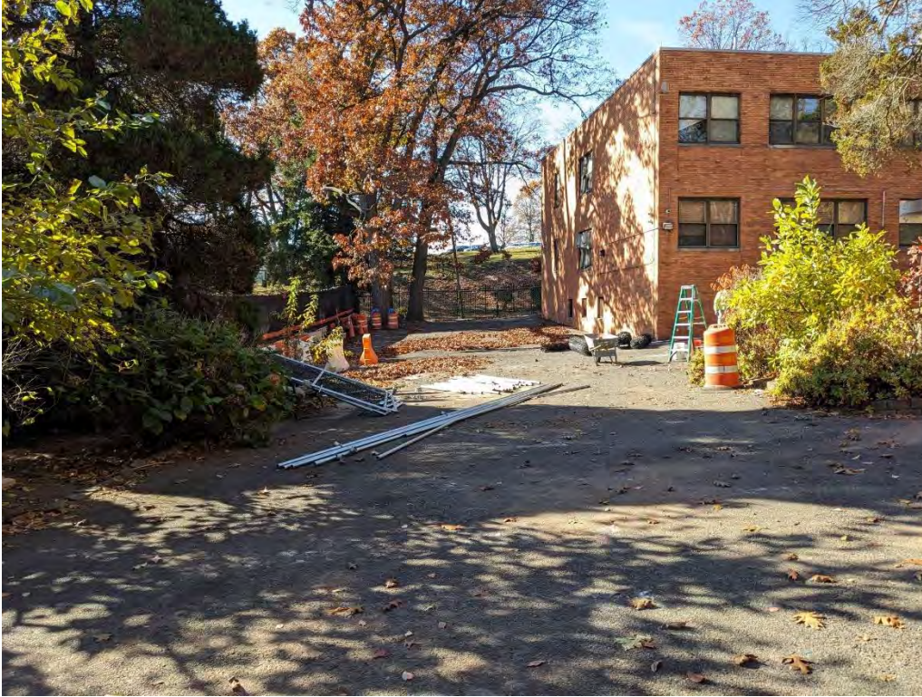
Photograph 9. The rear of the former high school. View looking southwest.
