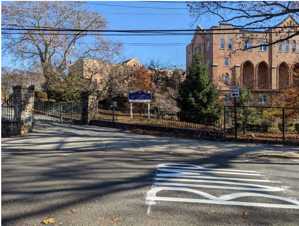
Photograph 1. The entrance to the St. John Villa campus from Cleveland Place. The former chapel building is on the right and the former elementary school building is in the far background. View looking east.
