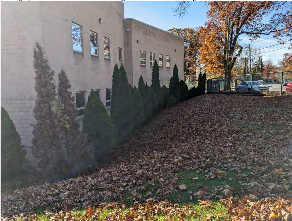
Photograph 10. The side of the former high school. View looking southwest.
