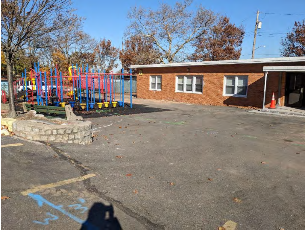
Photograph 11. The former childcare building and play area. View looking north.
