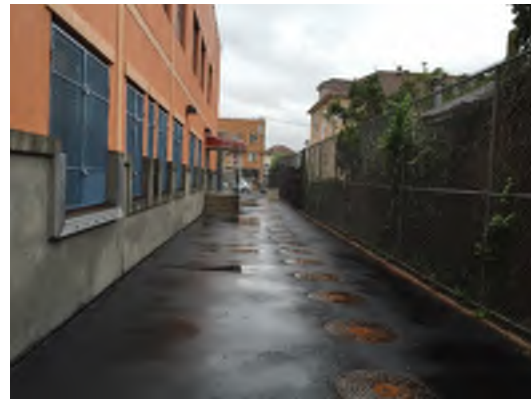
Figure 1: Reinforced Exterior Walls.
